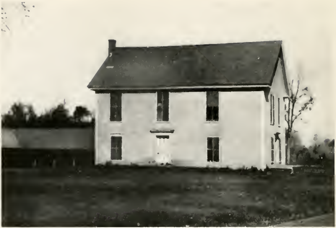
THE BAPTIST MEETINGHOUSE IN WEST CLARENDON, VERMONT, BUILT IN 1798. HORSE SHEDS IN THE REAR
